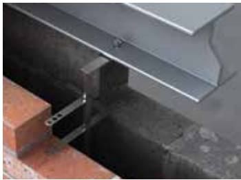
Offset head where there is no fixing directly above. Heavy-duty.
