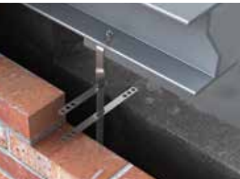
Used as a soffit fixed head restraint. Light-duty, twisted head allows for fixing a right angle to cavity.
